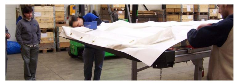
The curtain is fixed temporarily by screwing manually the nut on the screw facing the center line of the roof. This will put in place the curtain over the whole length of the roof.
